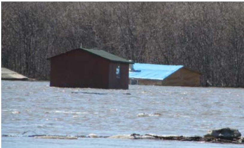
Cabins were uprooted and floated down the Peel River during 2013 spring flooding near Fort McPherson. Photo credit: David Cook
