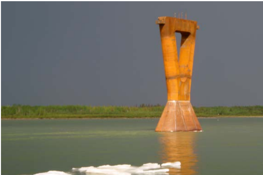
The Deh Cho bridge under construction. Photo credit: Kerry Wheler
