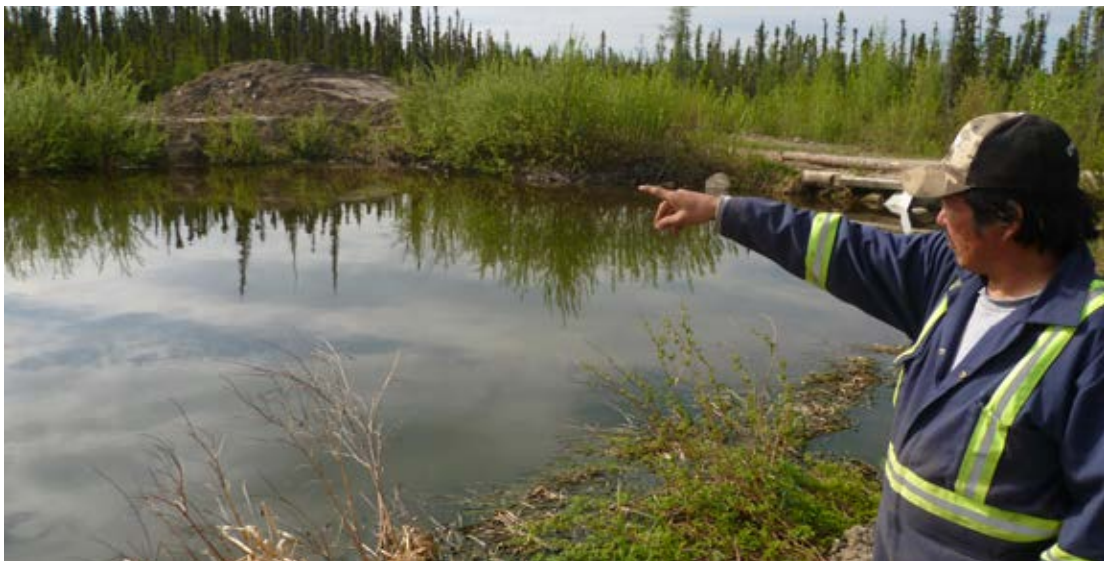
The foreman explains annual maintenance work needed to maintain berms at the wastewater lagoon, Trout Lake Photo credit: Christine Wenman
