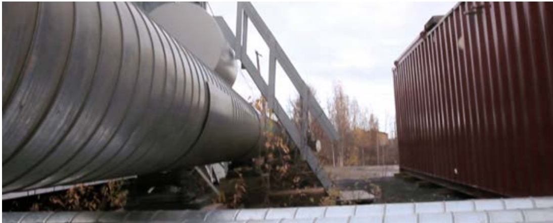
A pellet boiler in Fort McPherson provides district energy and with increased growth of Willows, biomass can now be harvested locally for energy. Photo credit: Davis Heels
