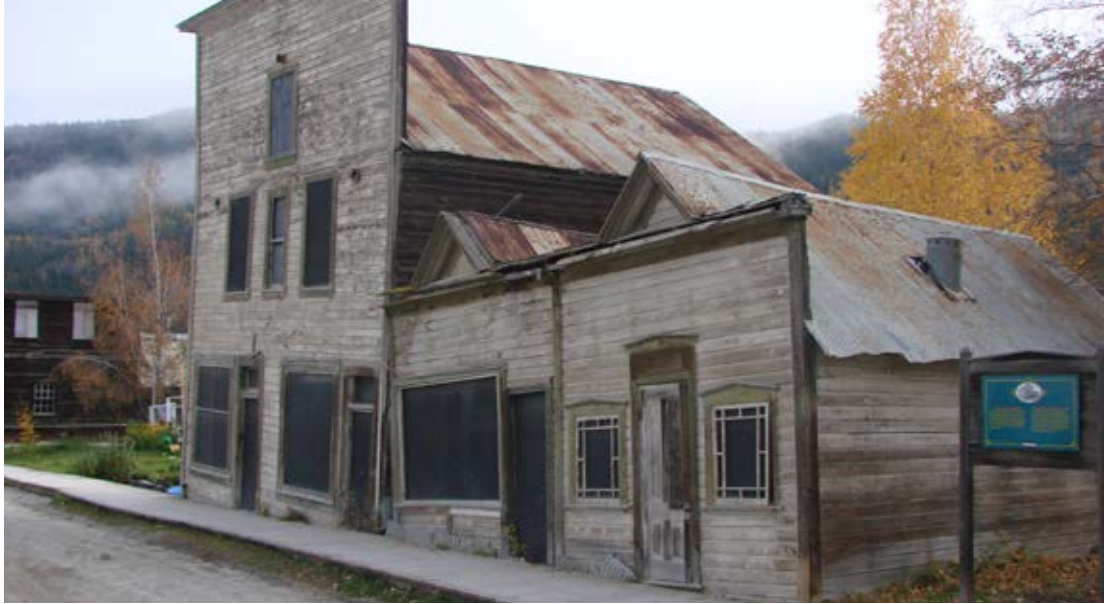
Permafrost affects bearing capacity and differential settlement as starkly illustrated in one of Dawson City, Yukon's iconic buildings.. Photo: Craig Scott
