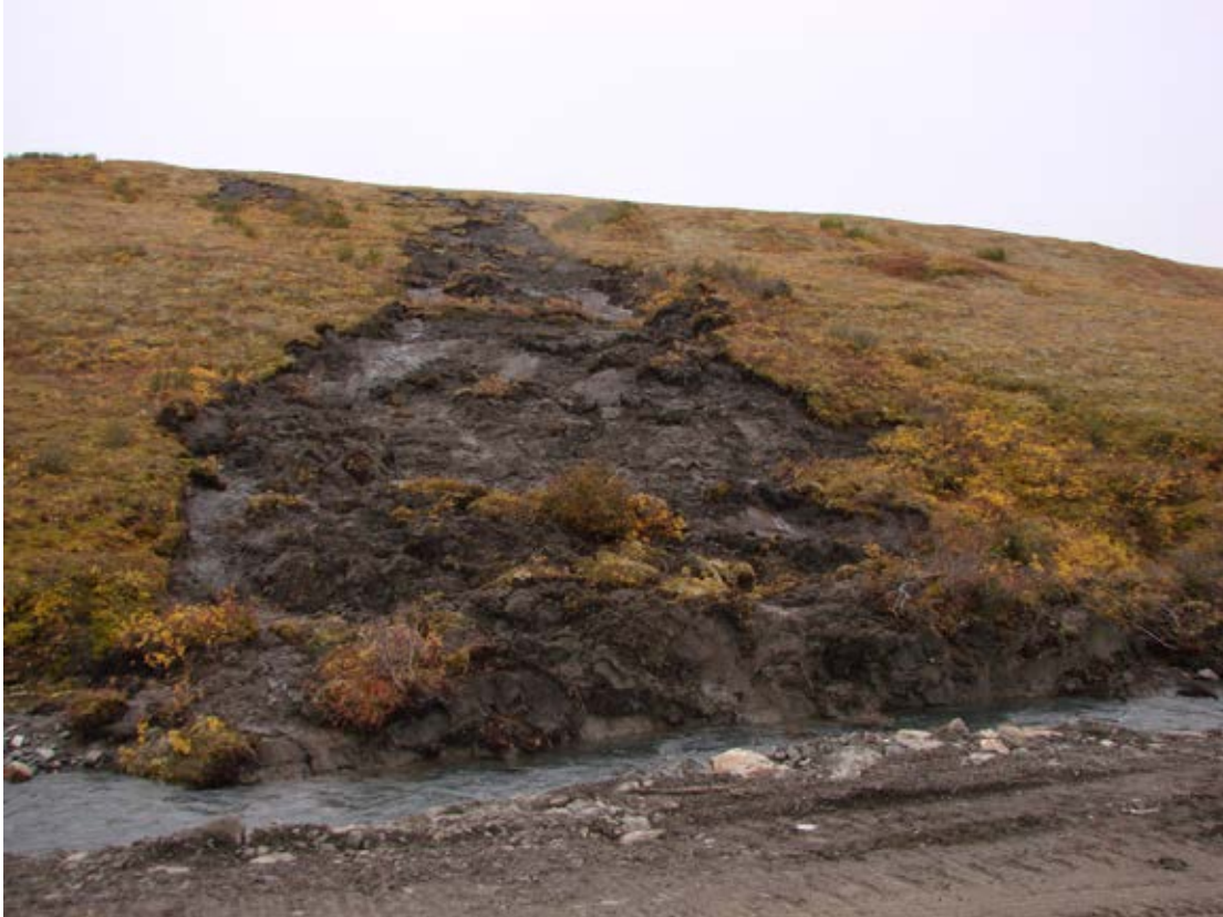
Small slump on the Dempster Highway. Photo: Craig Scott
