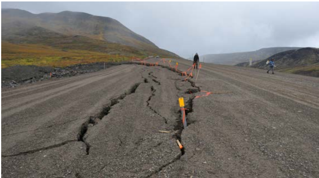
Frequent road maintenance is required on the Dempster Highway because of permafrost thaw and slumping. Photo credit: GNWT
