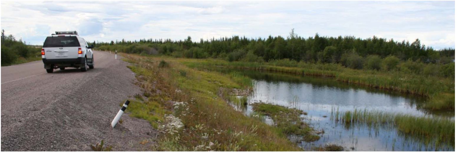
Photo 1-6. Elevated road surface on Highway 3. The tipped delineator (white and black marker) shows where the ground has moved and where the original surface was. Note that a 6:1 (less steep than shown here) side slope flattening close to water bodies is now recommended. NWT Department of Transportation, Highway 3 - Climate Change Vulnerability Assessment Final Report, Appendix B, 2011 .
