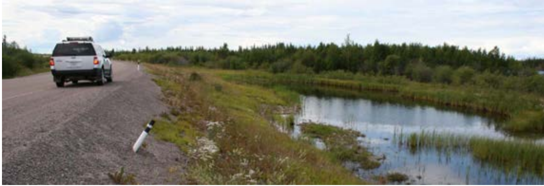
Elevated road surface on Highway 3. GNWT Department of Transportation. Highway 3 Climate Change Vulnerability Assessment . 2011.
