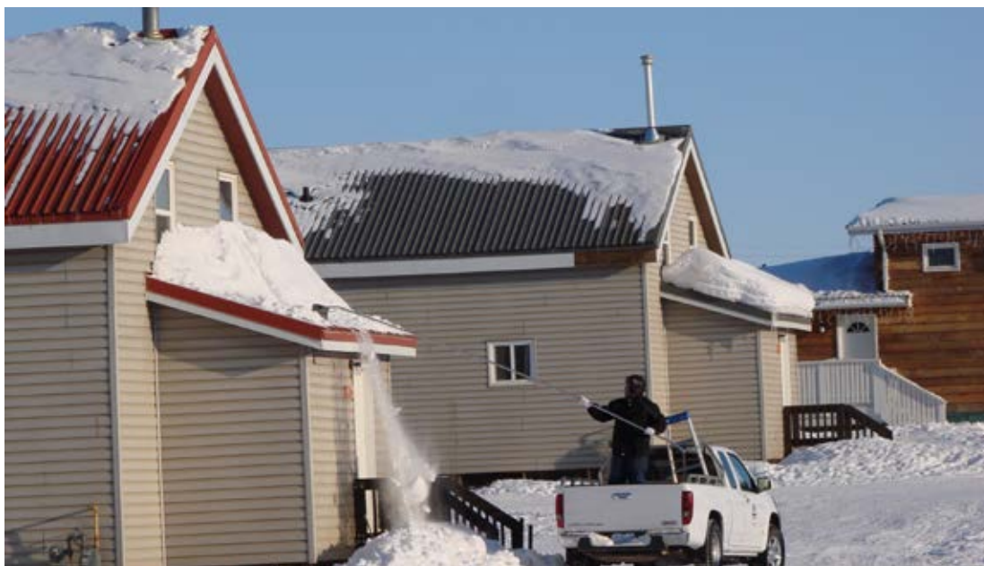
Clearing snow off roofs in Inuvik. Photo: Craig Scott
