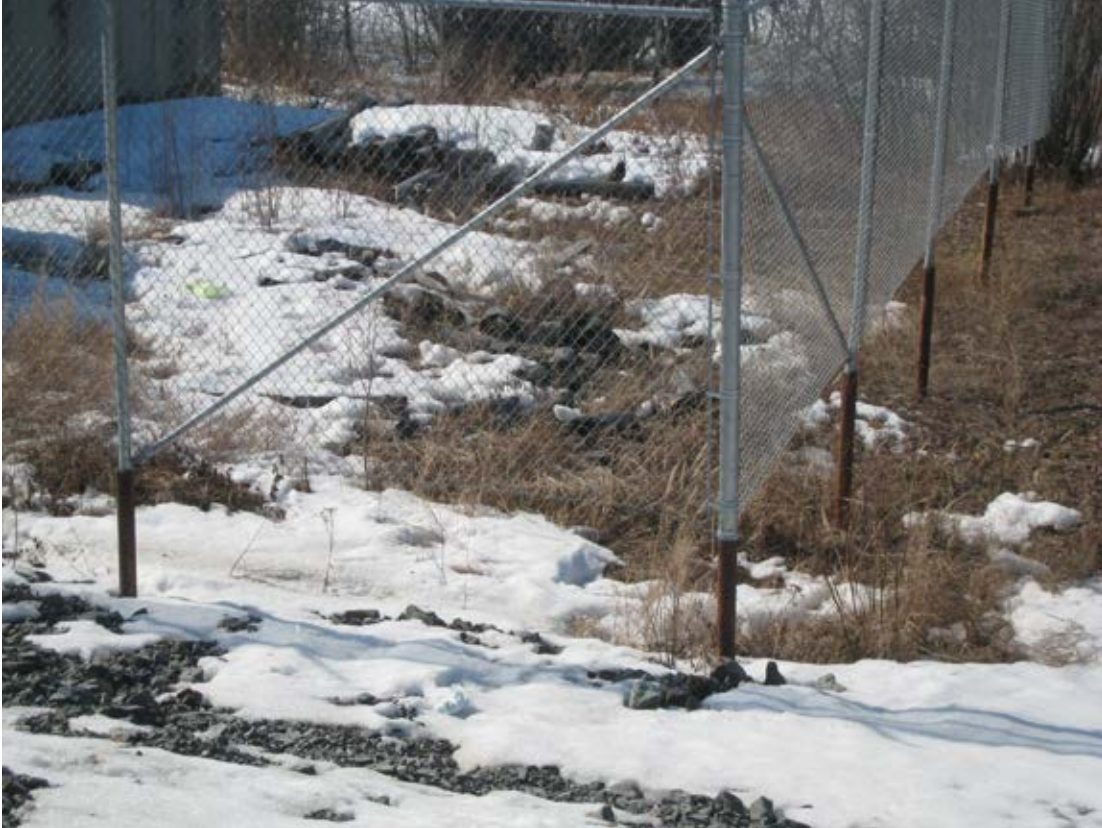
Frost heave lifting the fence. Photo: Ellen Pond
