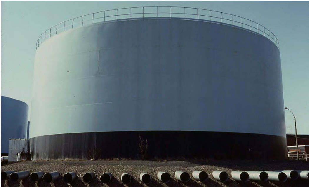
Figure A.7 Photo of a ventilated gravel pad beneath a storage tank, Inuvik, NWT (See Clause A.2.2.4. )
