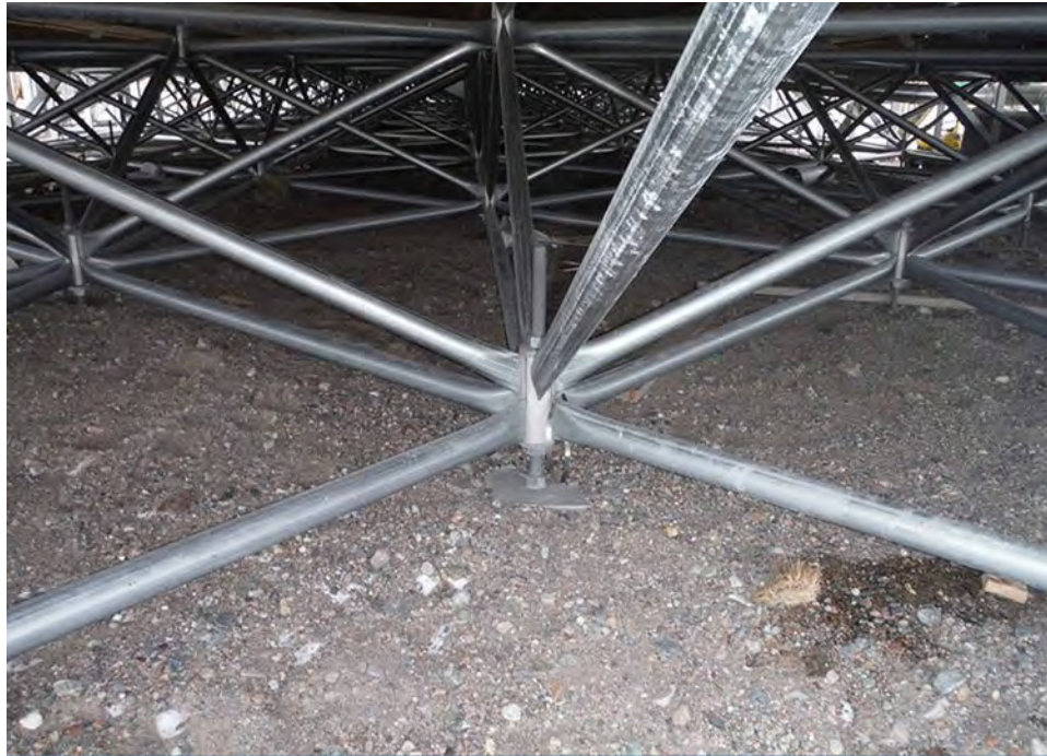
Figure A.3 A TRIODETIC® foundation (See Clause A.2.2.2. )
