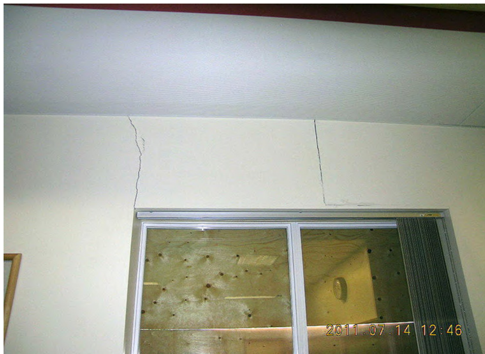
Figure B.12 Cracks above interior window of school in central Yukon (See Clause B.4.)
