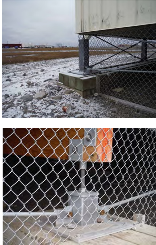
Figure A.2 Two photos of adjustable footings at ground surface (See Clause A.2.2.2.)
